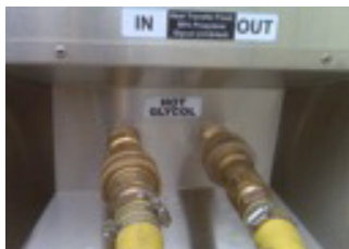
28: Hoses Connected to HD308 Unit
