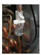
Thermistor attached to the refrigerant line.
